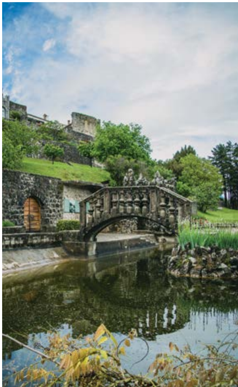
One of the most beautiful works of the architect Maks Fabiani is the Ferrari Garden in Štanjel. Photo: psgt_123/depositphotos.com
