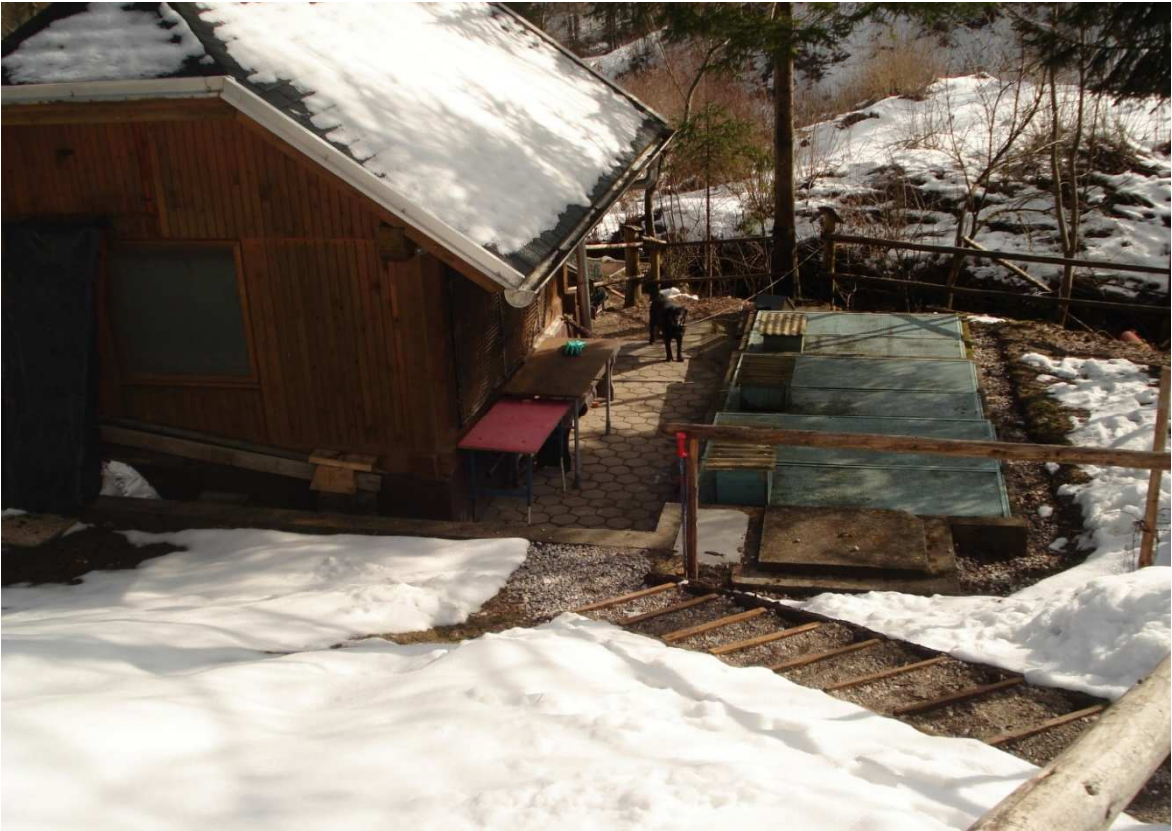
Photo 4 – Hatchery and 3 sequential concrete tanks
