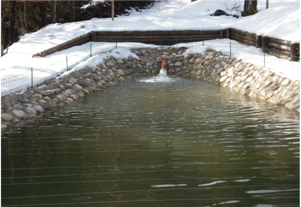
Photo 1 - Inlet to the concrete tank for brood stock
