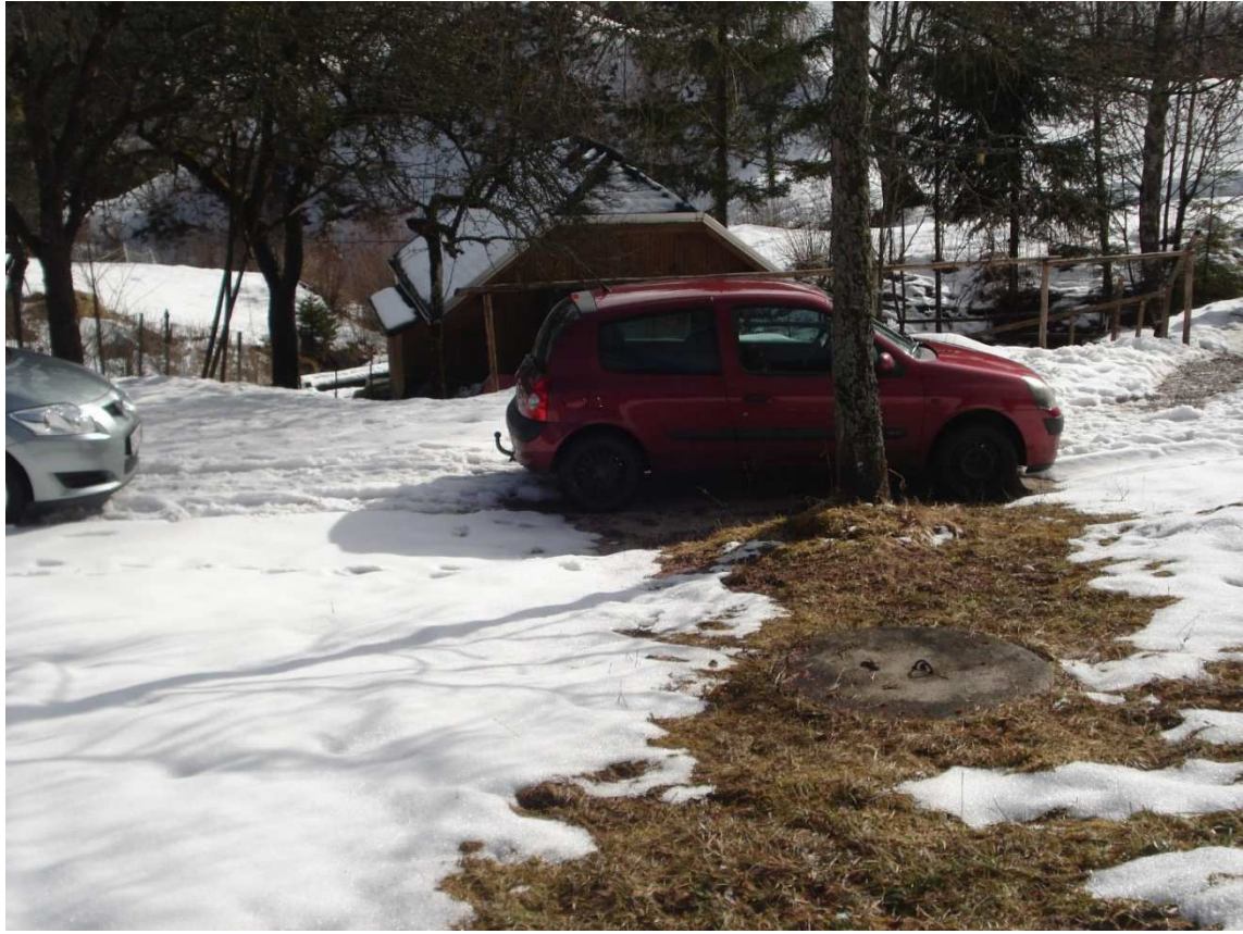
Photo 3 - water capture fort he hatchery and 3 sequential concrete tanks (concrete cover)
