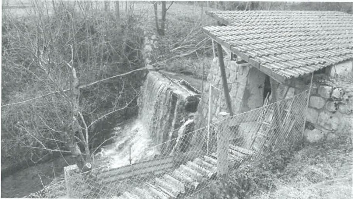
Okroglo spodnja pregrada 4,2m Photo 11 - dam (4,20m) - end of compartment
