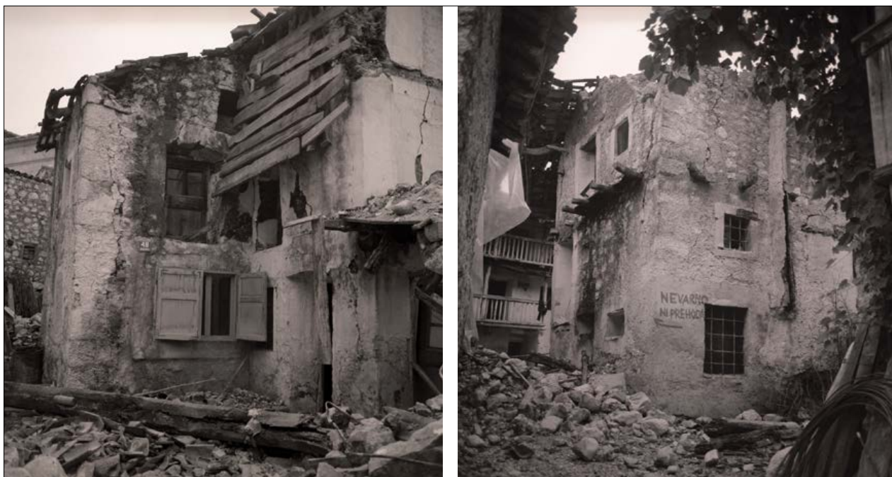
Sliki 2 a in 2 b: Velike poškodbe na starih kamnitih hišah v Breginju (© Ministrstvo za kulturo, INDOK center, J. Gorjup, 1976) Figure 2a and 2b: Heavy damage on old stone houses in Breginji. (© Ministry of culture, INDOK center, J. Gorjup, 1976)
