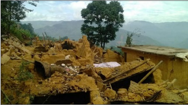
Slika 3: Zhoujiaping, po potresu 3. avgusta 2014 Vir: http://en.wikipedia.org/wiki/2014_Ludian_earthquake#/media/File:Zhoujiaping_after_Ludian_earthquake.jpg
