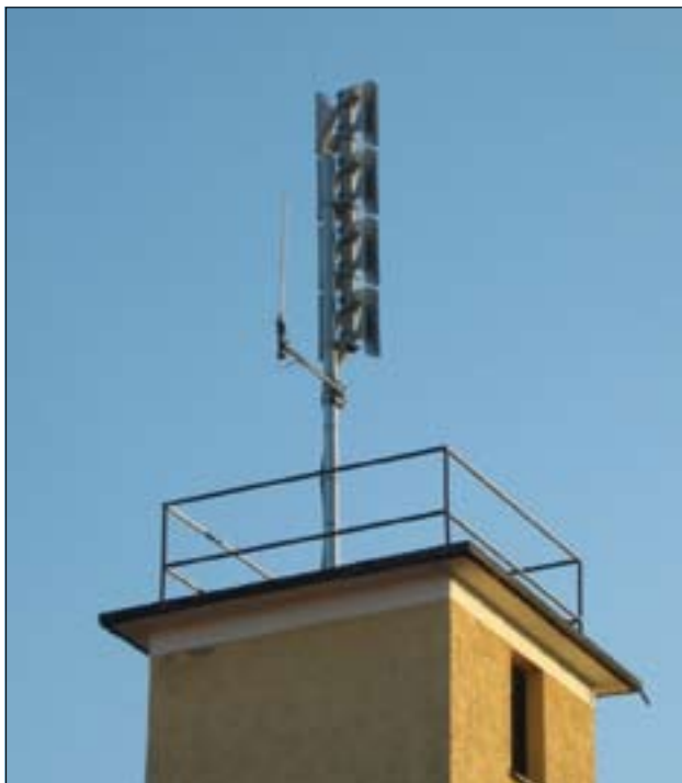
Slika 1. Nova elektronska sirena proizvajalca Sonnenburg Electronic AG Figure 1. New electronic siren made by Sonnenburg Electronic AG
