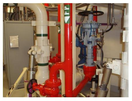
Figure 12: Fire insulation valve 28985 (the valve is located on the fire pipe for extinguishing reactor coolant pump No. 1)
