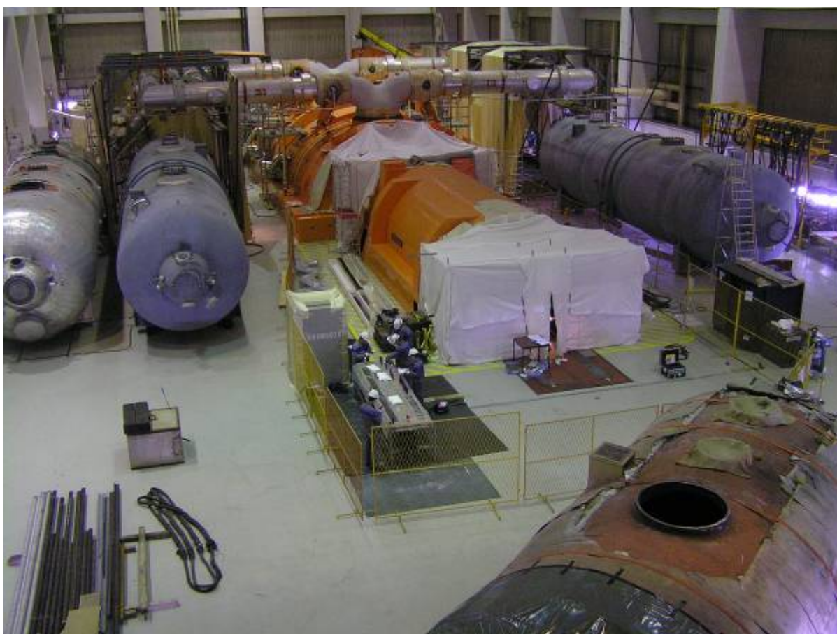
Figure 10: Two new moisture separator reheaters (blue color)
