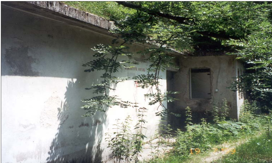
Figure 2.46: The outer walls of the barrack – placards and inscription "radioactive" were removed
