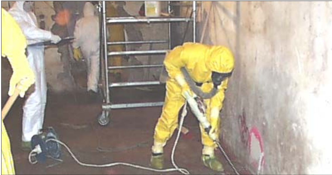
Figure 2.45: Subcontractor's staff during decontamination of the room, where radioactive waste had been stored
