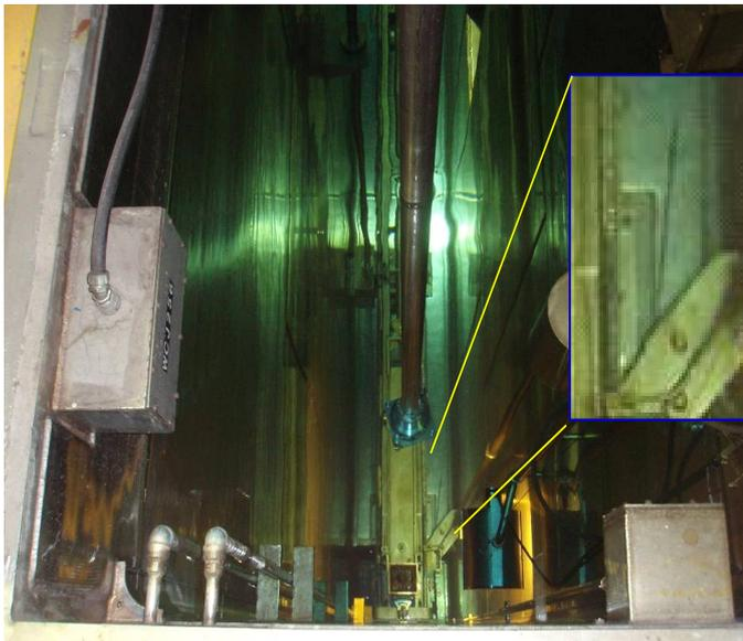
Picture 1: Part of a broken fuel rod at the bottom of the fuel transfer canal
