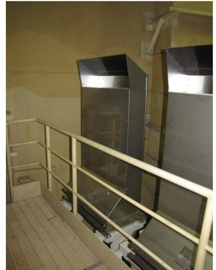
Picture 2: Installed PAR units
