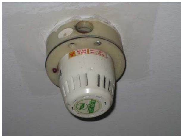
Fig. 2: Typical ICSD using 74 kBq of Am-241 installed in a shopping center in Ljubljana.
