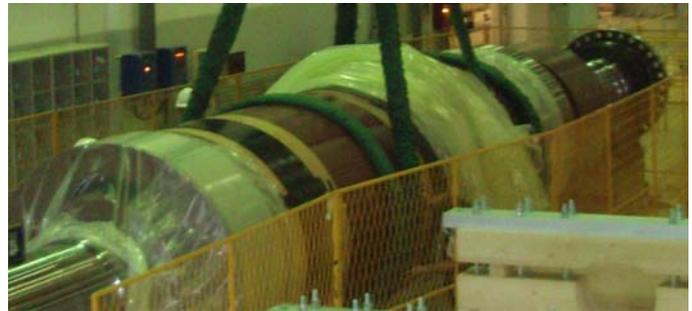
Picture 1: Rotor of the main electrical generator
