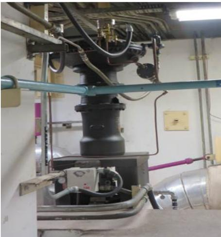
Integrated I/P converter together with positioner of the FCV-551
