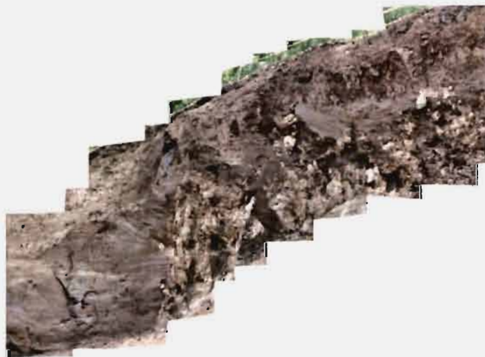
Fig. 8 . The Lithotamnian limestone is massive, fractured, weathered and intensively karstified. The contact with the “residual clay” is very uneven and corroded. There are isolated corroded fragments of limestone in the “residual clay”. The SW wall of the trench, between app. 1-8 m.
