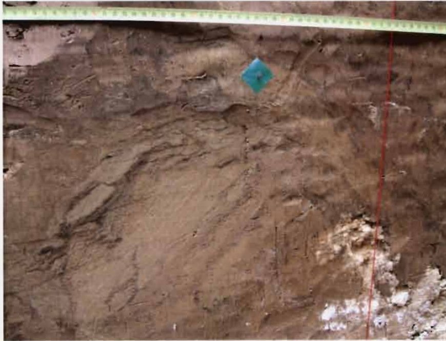
Fig. 35. The silty patches – ghost clasts and weathered limestone in the “residual clay”. The NE wall of the trench at 7.3 m.
