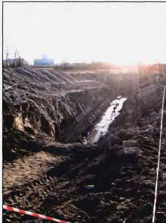
Figure 39. The view over the trench toward the WSW.
