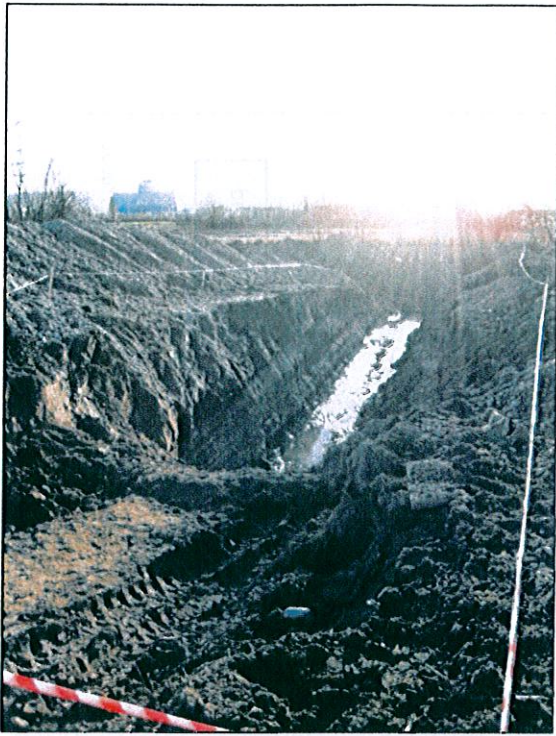
Figure 3. The view over the trench toward the WSW.
