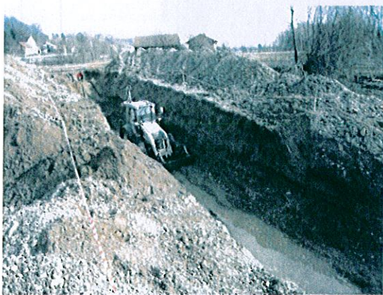
Figure 4. Groundwater inflow (app. 4 l/s) affected stability of trench wall.
