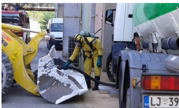
Figure 8: Precautionary measures at work involving powdery chemical substances
