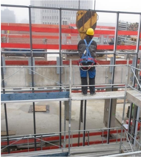
Figure 5: Proper use of personal protective equipment
