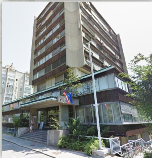
Figure 3: The headquarters of the Surveying and Mapping Authority of the Republic of Slovenia
