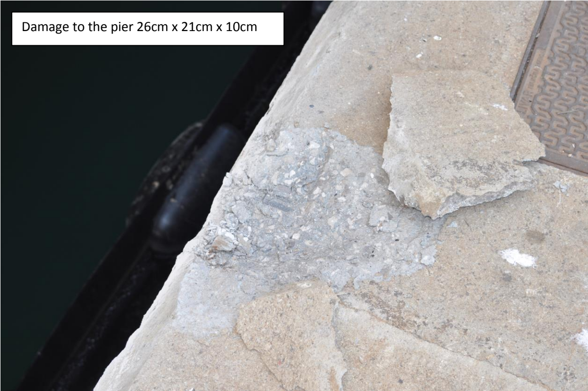
Picture 7: Damage to the pier
