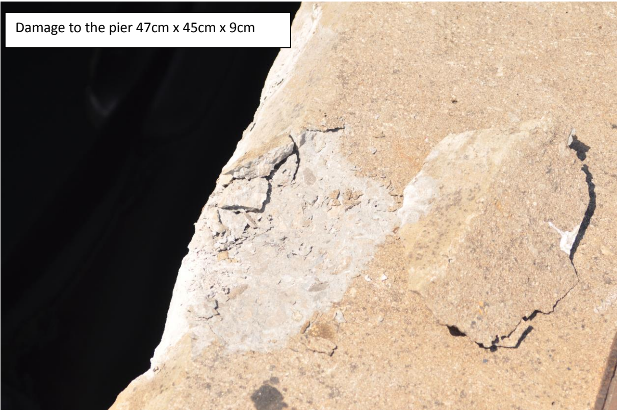
Picture 7: Damage to the pier
