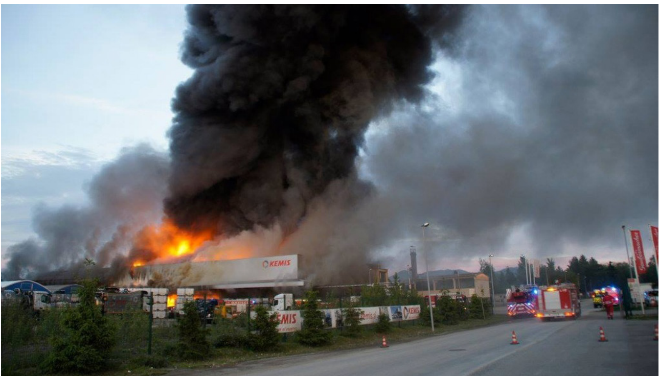
The Fire at Kemis
